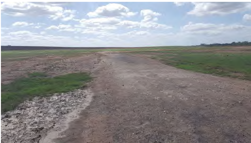
Figure A4 – Sheet erosion at MRP 41
